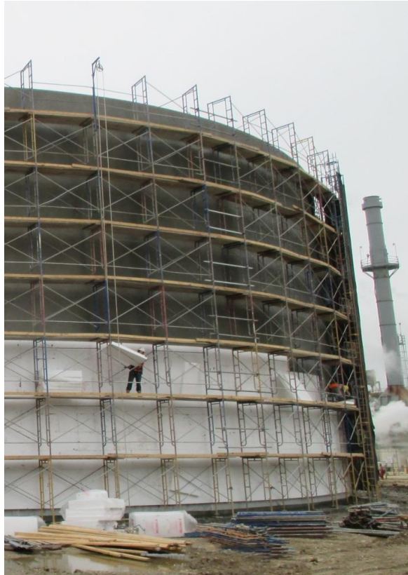
Polystyrene board epoxy bonded to the exterior wall
