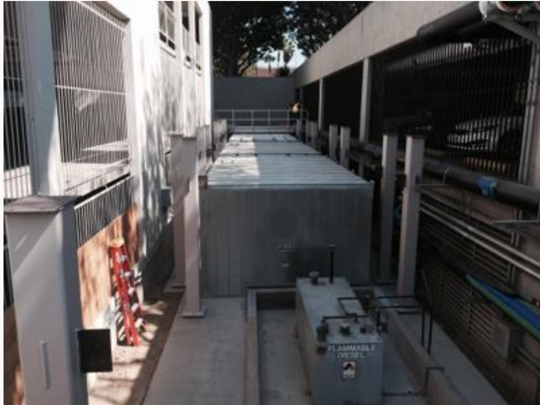
Molina Healthcare Long Beach, CA (10) Internal Melt Tanks 5,900 Ton Hours
